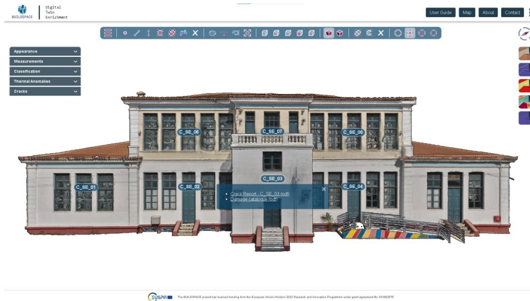
Figure 67. Cracks annotation example
